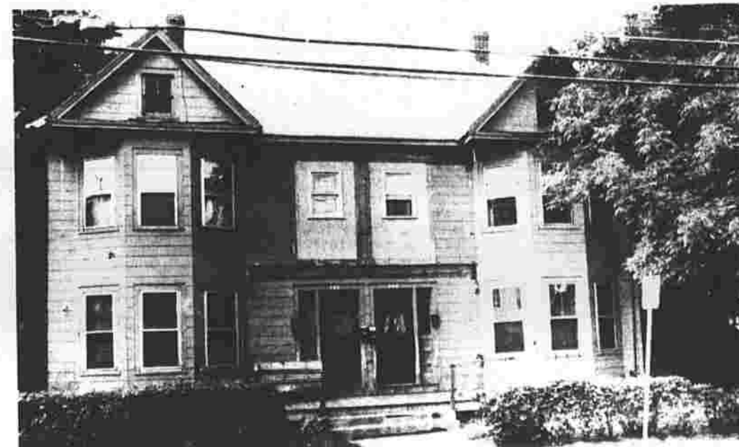
The landlord of this multi-dwelling unit at 124-126 Spruce St. has been ordered to correct several housing violations, including faulty plumbing and electrical systems.
